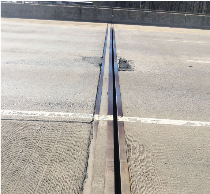
PHOTO 1 Description Bent 1 joint seal missing. Common bent 5.
