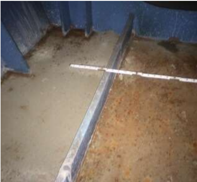
PHOTO 1 Description Girder 4 at first bulkhead back active rust with moderate pitting to bottom flange and lower web.
