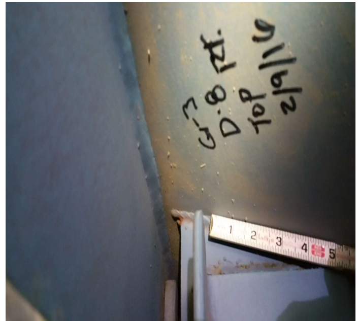
PHOTO 9 Description Girder 3 diaphragm 8 back right side. New crack in the weld at upper diaphragm.
