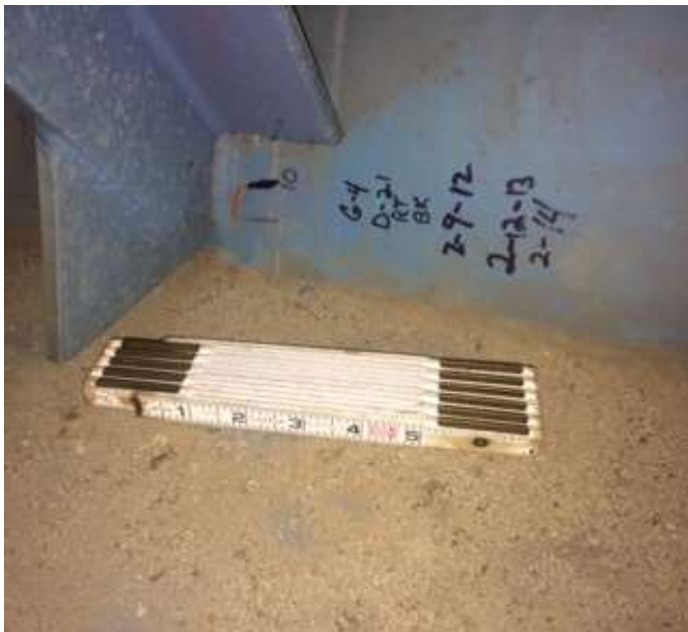
PHOTO 1 Description Girder 4 diaphragm 21 back crack in the web. No change.
