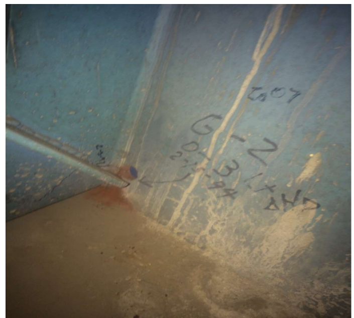
PHOTO 10 Description Girder 2 diaphragm 3 crack in the weld. No change.
